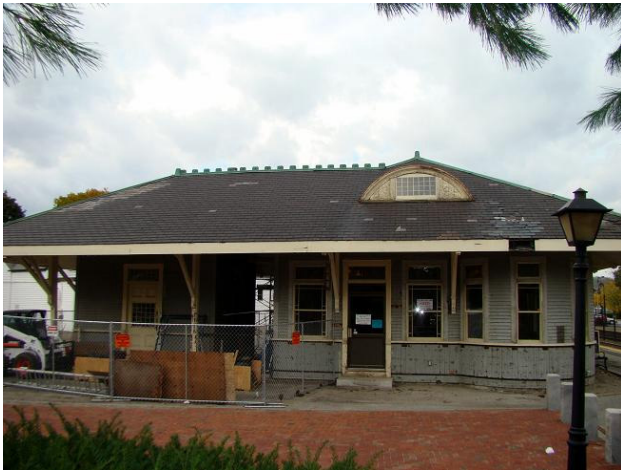
Renovation is in progress at the historic West Concord Depot
