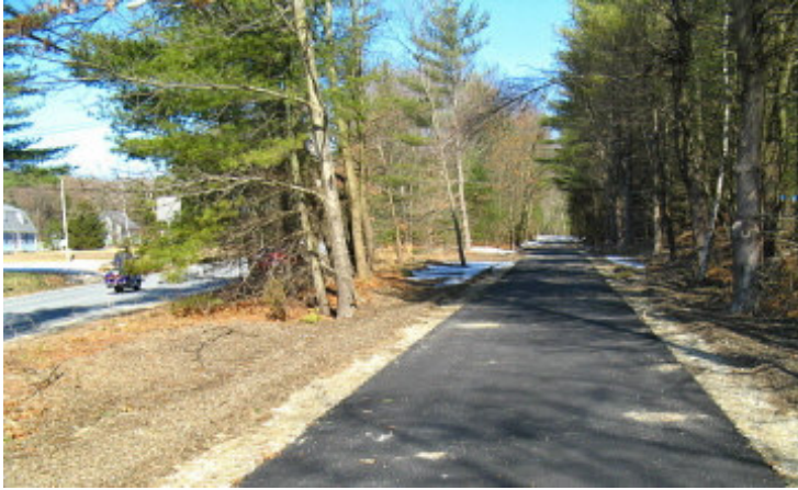
New pavement anticipating spring at Rts. 225 & 27 in Westford
