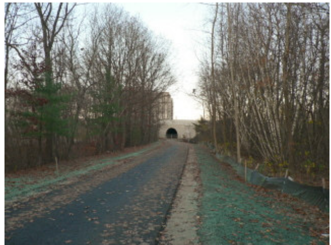
Binder course and seeded slopes in Chelmsford Cross Point Towers can be seen beyond the Rt. 3 tunnel
