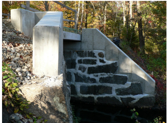
Part of the Phase 1 progress, a reconstructed bridge in Chelmsford has new concrete wingwalls and deck on pre-existing repointed granite abutments. Railings and curbing will be installed after the trail surface is completed.
